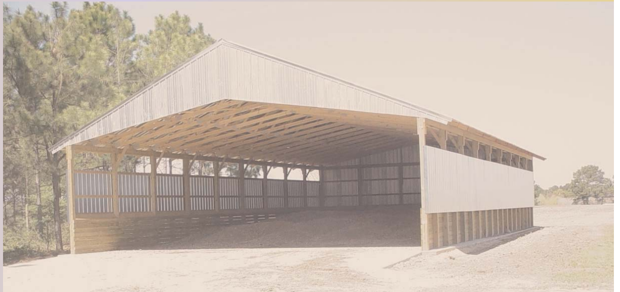
This new stackhouse will prevent harmful nutrients from getting in the water supply of Ware County.
