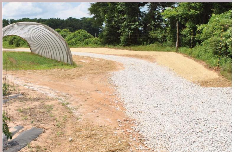
Bentoski installed critical area treatment. The road was graded and shaped and the ditch around the high tunnel was shaped to have a flat bottom to establish vegetation. This not only controls erosion but makes maintenance easier allowing the ditch to be mowed. This is a certified organic farm so weed control is mechanical.
