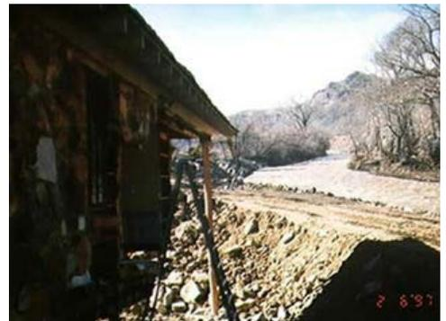
A constricted river channel caused the raging flood water to find a new path, carving a gorge under this house and carrying away another house just downstream
