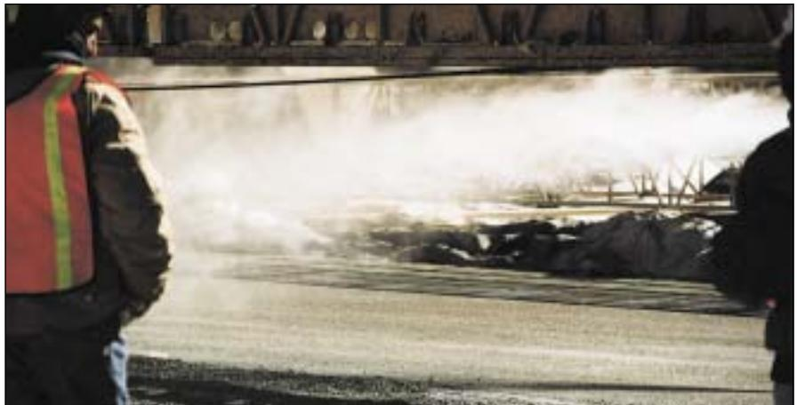
Above: When concrete mixes with water-cement ratios of less than 0.40 are being used, it's important to ensure that no mix water evaporates. Here, the contractor is fogging the air with a pressure washer while concrete is being placed. Below: Cotton mats are increasingly being used for wet curing. On the Wacker Street project in Chicago, cotton mat placement followed about 100 feet behind concrete placement.
