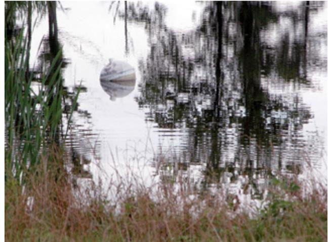
**The pipe in the pond is connected to a float which keeps the pipe about three feet below the surface of the pond.**
