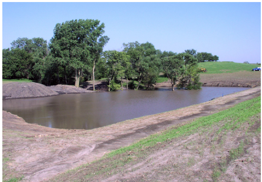
A newly constructed grade stabilization structure, completed in 2007, in the Hacklebarney Watershed with trees in the background that provide habitat for wildlife.
