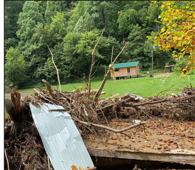
Debris damage after a severe rain event in Kentucky.
