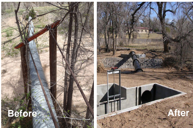
This RCPP project is bringing together partners to repair acequias, like this one near Nambe, N.M. Photos by Rey Adame, NRCS.
